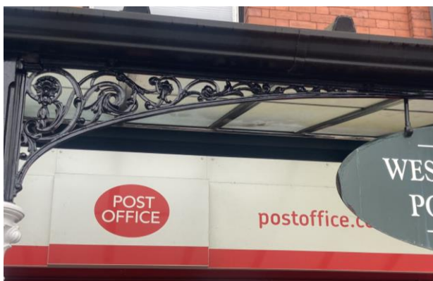
The replacement aluminium spandrel firmly secured for the future
