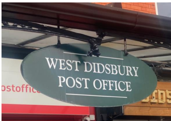
One of the resin spandrels on the point of disintegration
