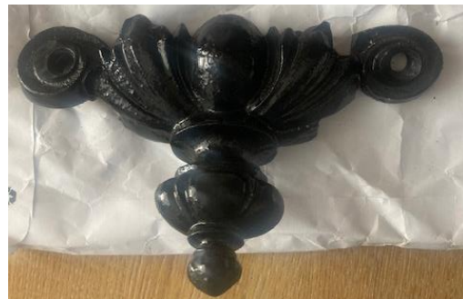
One of the ornate spandrel joiners to be found at the apex of each arch
